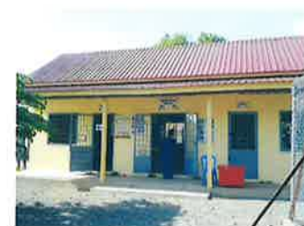
Health Post construction
